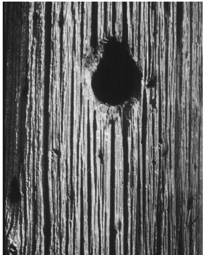
Figure 1.9 Woodpecker cavity in a utility pole. These holes allow water, fungi, and insects to enter the wood, accelerating deterioration.
