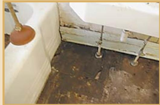
Leaking showers and sink quickly rotted the wood subflooring in this bathroom.
