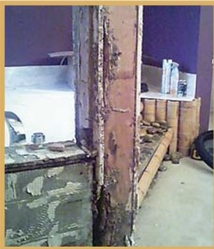
Leaking water and poor showering habits destroyed this supporting wood stud next to the bathtub.
