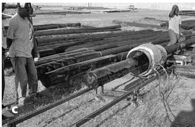
Figure 2.15 Typical barrier wraps for round and rectangular sections. From (a) http://www.postprotector.com ; (b) http://www.pplfieldliners.com/users.htm ; (c) http://www.pplfieldliners.com/users.htm ; (d) Barnes et al. (2009).
