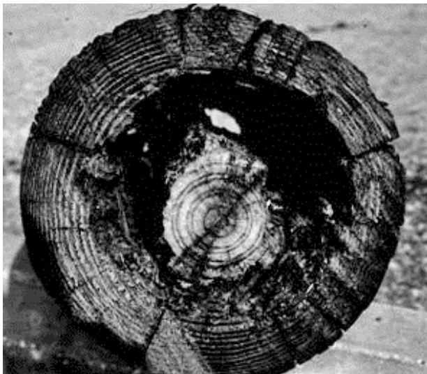
Figure 2.1 Typical core rot caused by fungi entering through a check across the well-treated shell into untreated wood.
