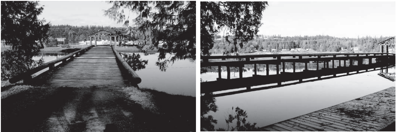
Figure 9.16 Seabeck Lagoon bridge, located in Seabeck, Washington, on Hood Canal.
