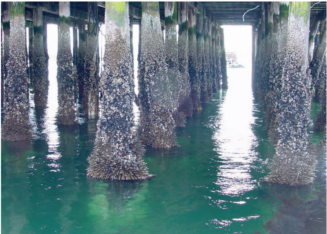
Figure P1. Creosote-treated piling supporting the Fort Ward pier and wharf in Washington contained over 60 invertebrate species on the low intertidal and subtidal portions of these piling. Barnacles were highest on the piling, followed by a community dominated by mussels, which transitioned to anemones and plume worms at low intertidal and subtidal elevations.
