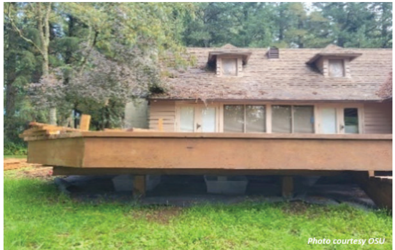
Rainwater runoff collected from under the deck was analyzed for copper concentrations. After initial dispersion of residual preservative from the wood's surface, the samples showed copper levels well below 1 ppm. Copper concentrations in soil samples taken beneath and downslope from the deck were indistinguishable from upslope samples and well within the normal range for the area.
