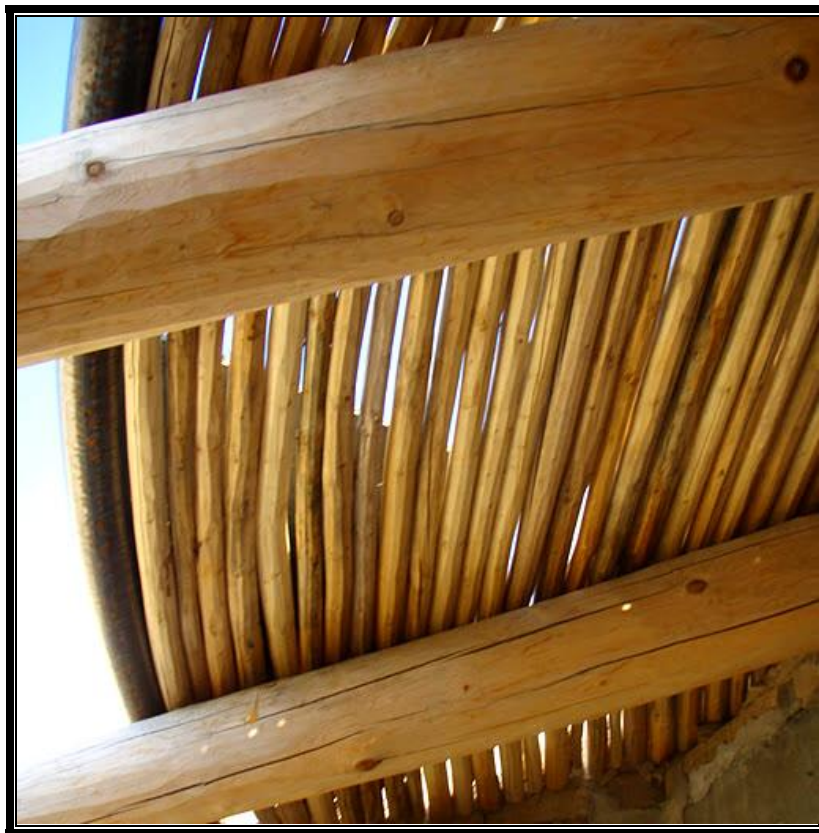
Figure 5 – Picture of a Latilla and Viga Roof
