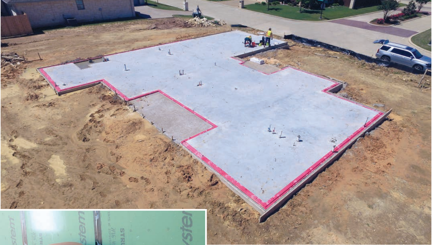
Peel-and-stick flashing moisture/termite barrier (left); Photos: Polyguard undersill moisture/termite barrier (above)
