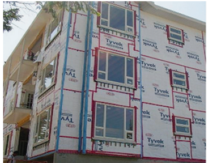
Continuous air barrier Photo: RDH Building Science
