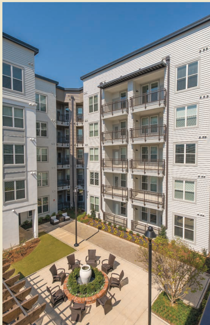
Clearance between landscaping and the structure allows for easy inspection
